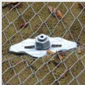
Examples of the system claw plates supplied by the mesh manufacturers, which are fixed using TITAN spherical collar nuts.
