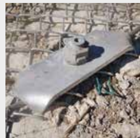
Examples of the system claw plates supplied by the mesh manufacturers, which are fixed using TITAN spherical collar nuts.
