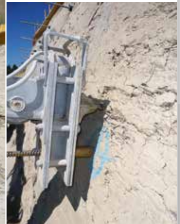
Exact alignment of the drilling rig at the drilling position.
