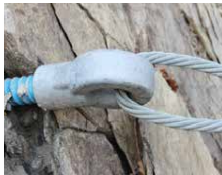
Track barrier with protection against rockfall made from ISCHEBECK hollow steel bars fitted with eye bolts for hexagonal chain-link fencing.
