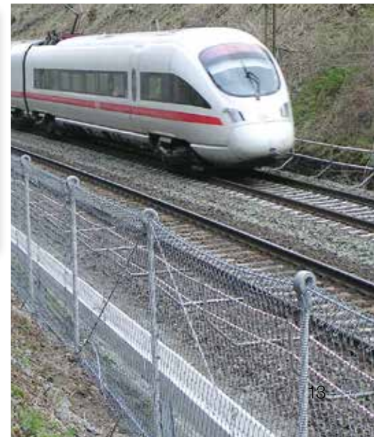
Track barrier with protection against rockfall made from ISCHEBECK hollow steel bars fitted with eye bolts for hexagonal chain-link fencing.
