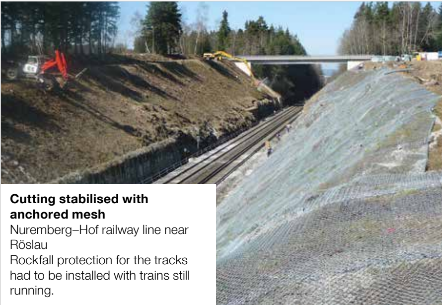
Laying the high-strength wire netting
