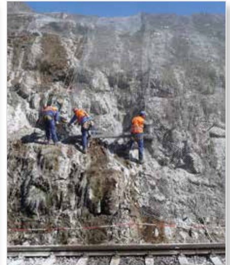
Laying the high-strength wire netting
